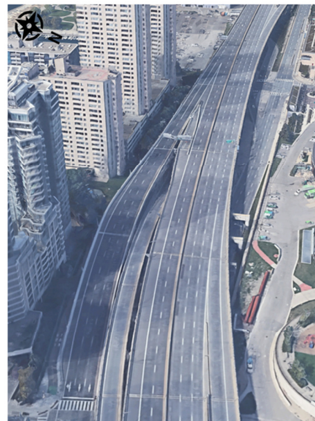
2 Gardiner Expressway WB York St On-ramp – Spadina Ave Off-ramp
