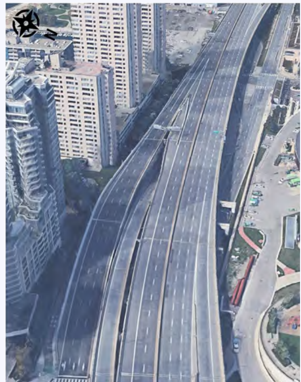
Gardiner Expressway WB York St On-ramp - Spadina Ave Off-ramp
